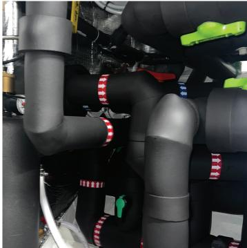
Marine Air completed, Castañeda used AP/ArmaFlex insulation, ArmaFlex Insulation Tape, and ArmaFix EcoLight pipe supports to successfully insulate hard-to-reach pipes in tight quarters. "I rely heavily on my training for these tricky installations below deck. Armacell provides not only superior customer service, but also industry trusted training. I have gained knowledge from Armacell by attending their AQIP training and taking Armacell Academy training classes."
