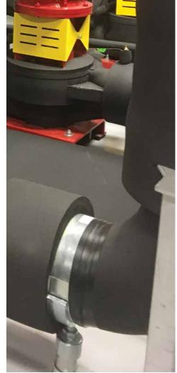
New chiller equipment insulated with ArmaFlex (installation not final)
